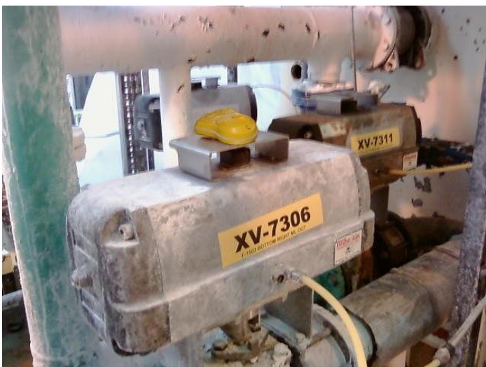
Eltav's Valve Device (VD) installed on an Actuator
