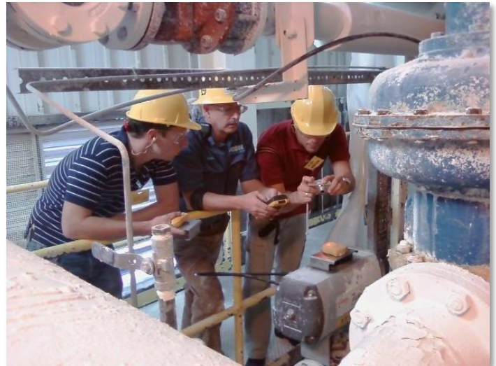
Configuring a Valve Device (VD) using the Eltav Operator's Device (OD)
