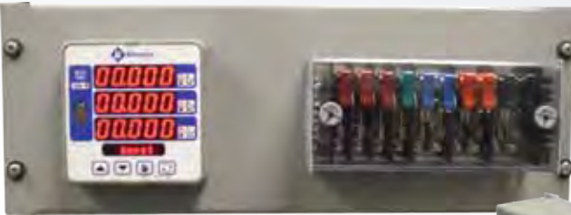
Front and rear views of M571 and remote display mounted to panelboard
