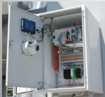
Custom enclosure with Bitronics 70 Series instrument and peripherals
