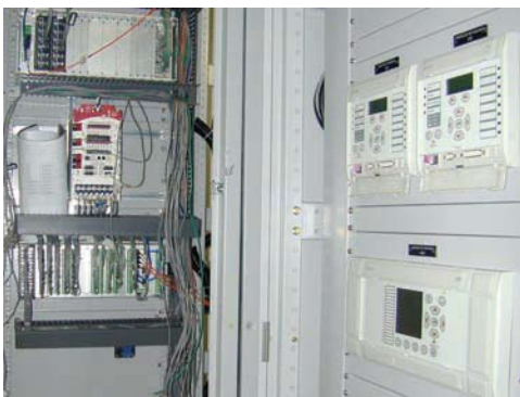
Beta testing facility in São Paulo, Brazil
