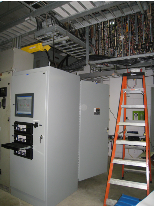
Photographs from the installation and commissioning of the first two RTU assemblies, the first requiring four days and the second requiring three days. Note overhead interconnection wiring.
