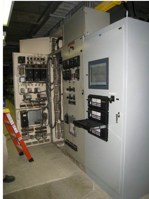
Photographs from the installation and commissioning of the first two RTU assemblies, the first requiring four days and the second requiring three days. Note overhead interconnection wiring.
